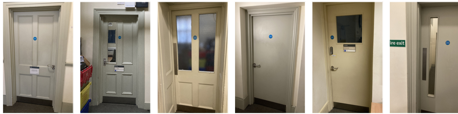
4 PANEL, SOLID DOOR 4 PANEL DOOR WITH ONE VISION PANEL 4 PANEL DOOR WITH TWO VISION PANEL BLANK SOLID DOOR BLANK SOLID DOOR WITH SQUARE VISION PANEL BLANK SOLID DOOR WITH LINEAR VISION PANEL
