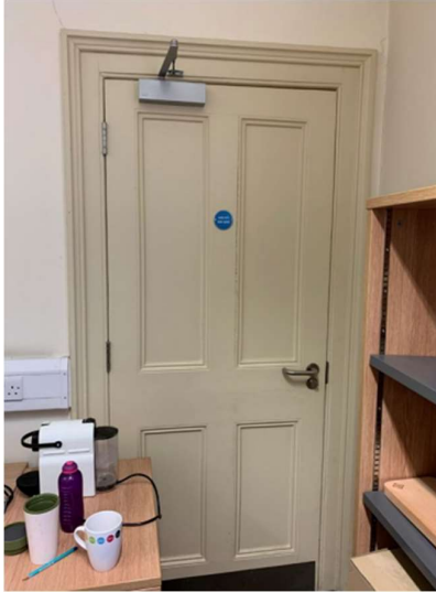
Figure 4 - Photograph of an example doorset to be sealed (Floor 2)
