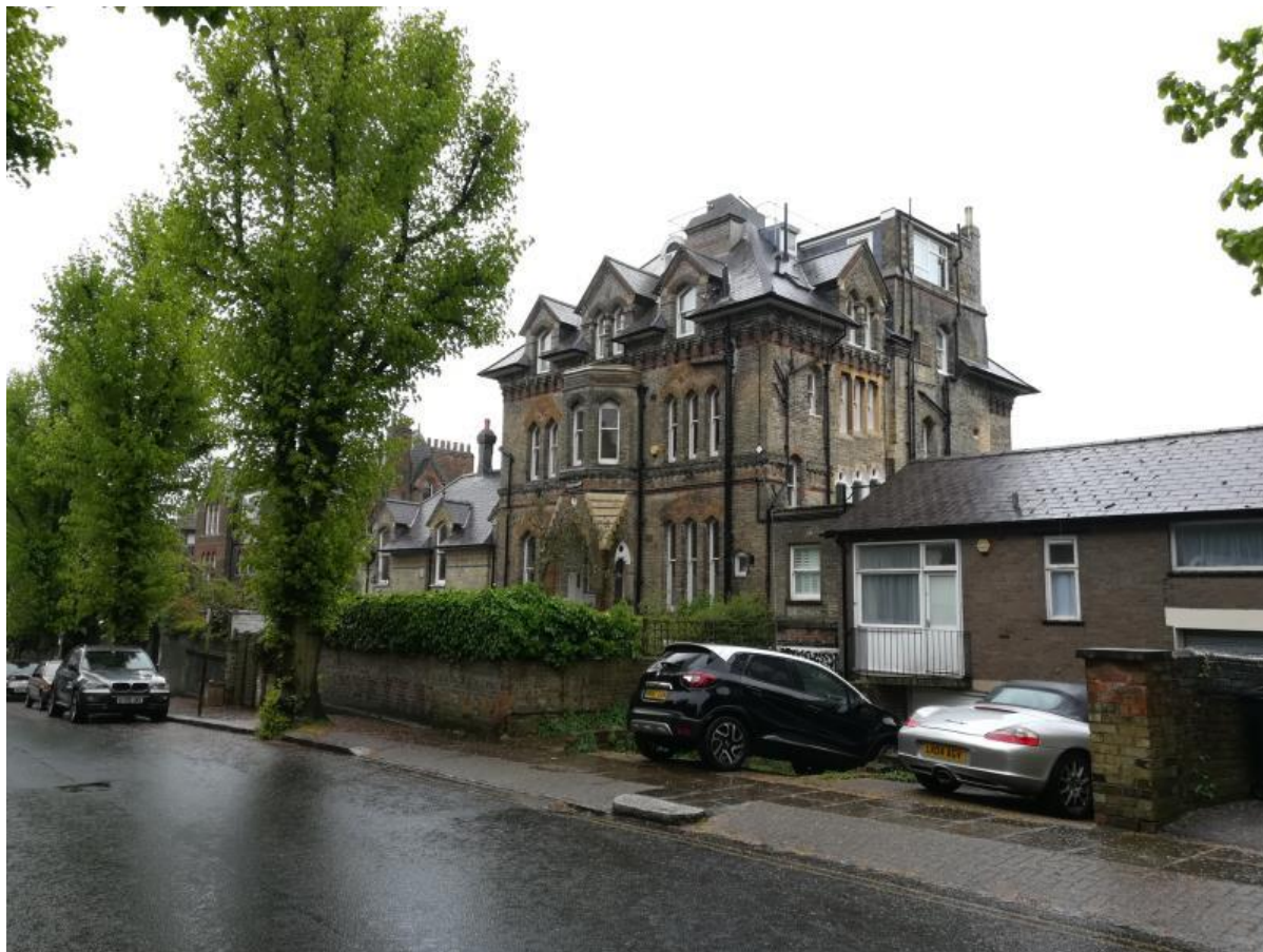
Photo 1: Looking south-west towards the Application Site (to the right) from Lyndhurst Terrace.
