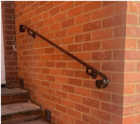
Figure 1 – Black metal railings fixed to masonry
