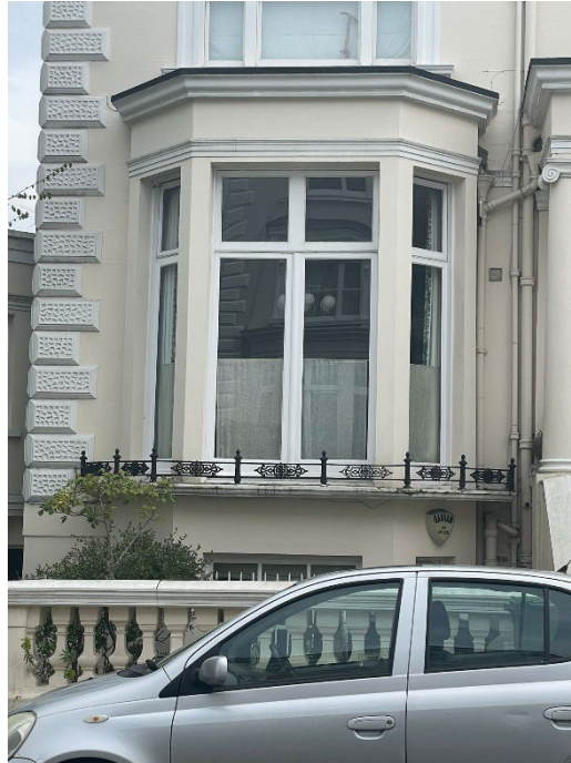
Figure 3 – Black decorative railings to front bay window
