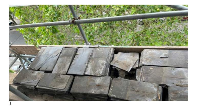
Original roof slates that have been kept for the roof repair and re-covering. The slates that were missing or broken will be replaced by reclaimed Welsh blue roof slates of the same size. Comparative photos included in the following photos.
