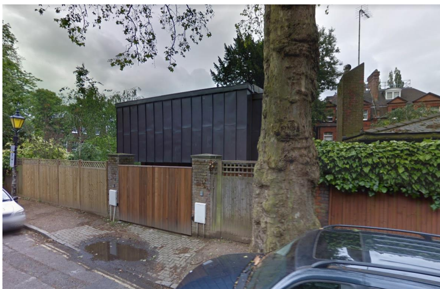
Figure 7. View of Ancillary building at 11 East Heath Road from Well Road (Google Maps)
