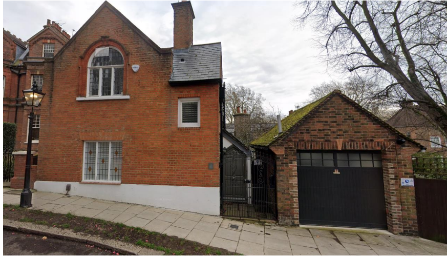
Figure 14. Entrance to No. 5 Well Road
