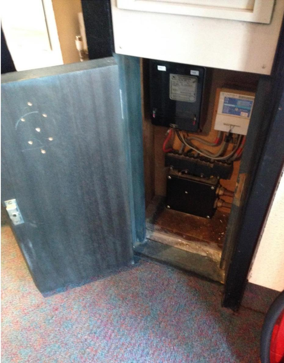
**Photograph 2: Inside of Typical Electricity Meter Enclosure**
