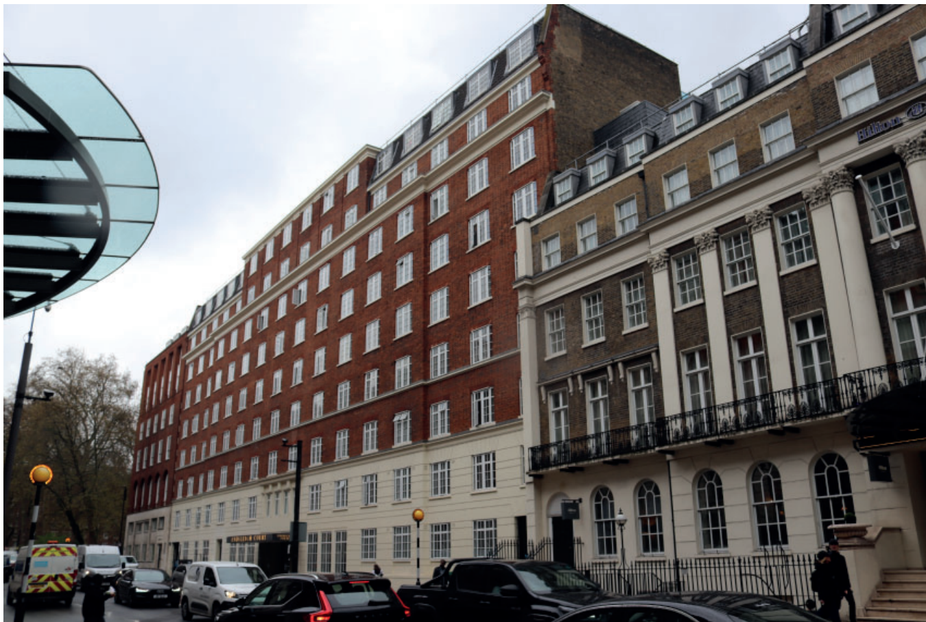
Fig. 11. Hilton Hotel (right hand side) with Endsleigh Court
