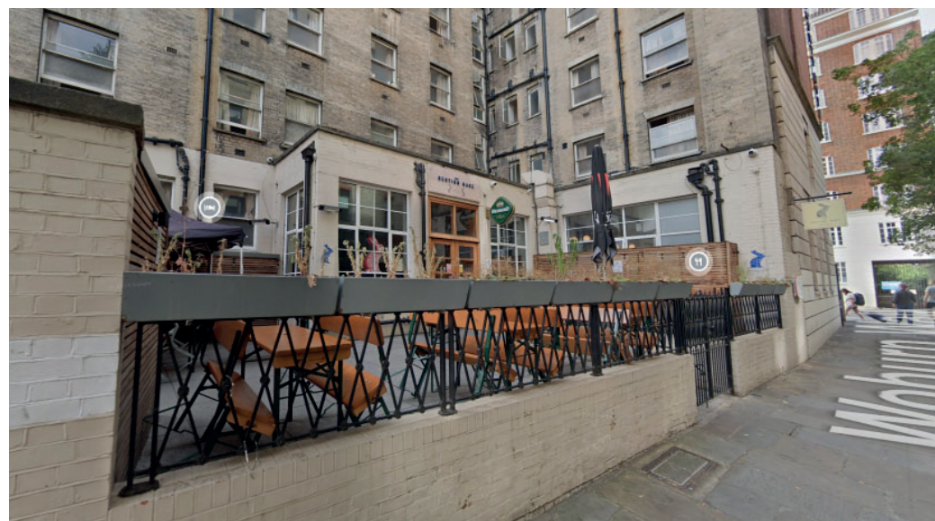
Fig. 14. Woburn Walk terrace and side elevation ©Google Street View 2023
