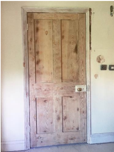
Internal Four-Panelled Doors
