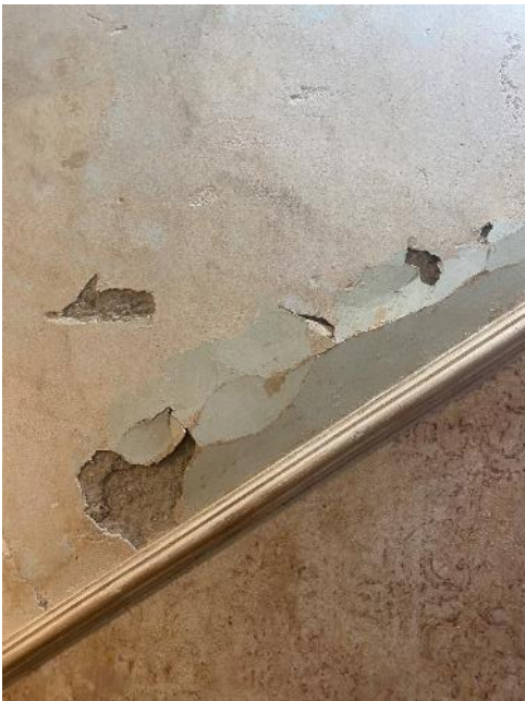
Loose and Damaged Plasterboard
