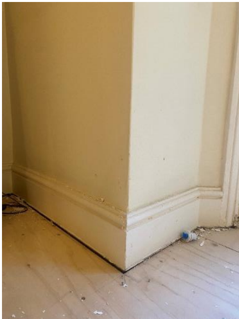
Lower Ground Floor Non-Original Skirtings Throughout
