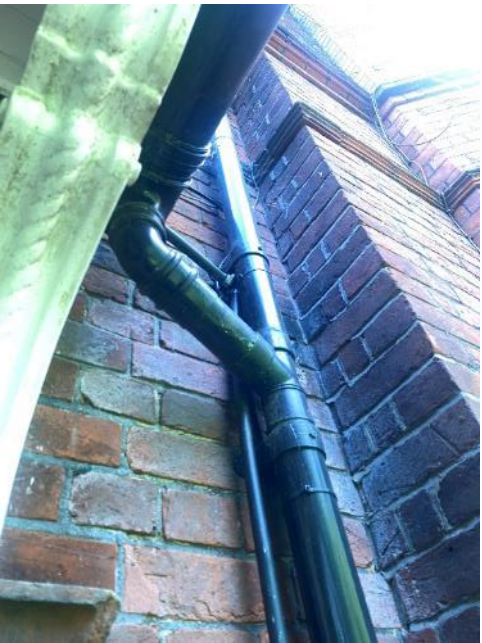
Non-Original Black UPVC Soil Vent Pipes
