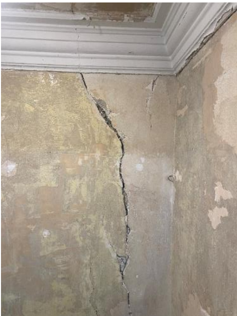
Prominent Cracks in Plasterboard
