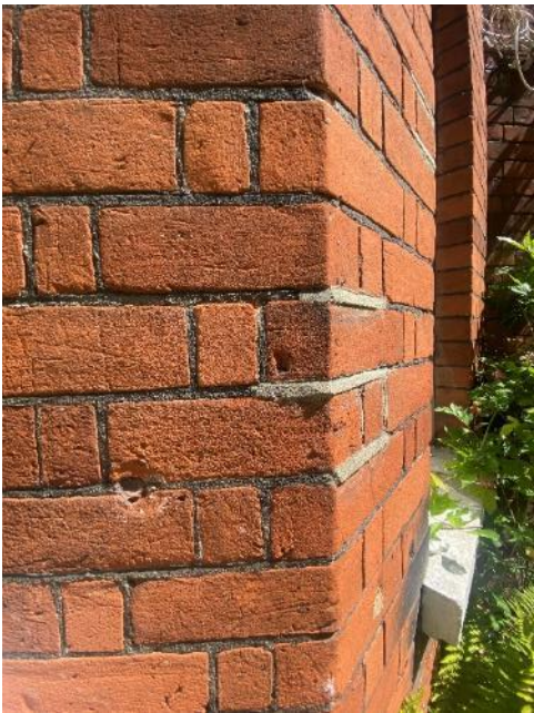
Masonry Wall – Front Façade Showing Poor Repointing Works
