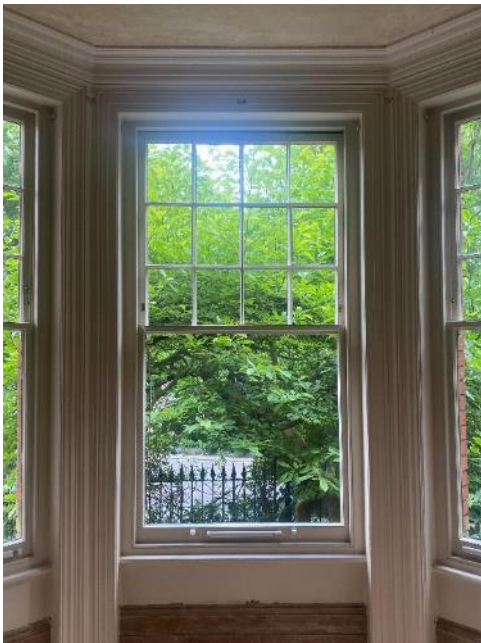
Single Glazed Timber Sash Windows With
