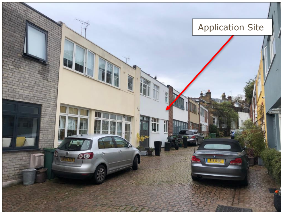
Figure 1: Photograph of 15 Belsize Park Mews and adjacent buildings
