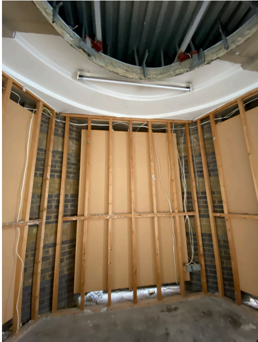
23.07.13 - Interior image with view towards original brickwork that was concealed behind a studwork wall. This being brick and not blockwork further illustrates the original intention to have this as the main opening onto Seven Dials. Reveavling original plans to have this as an exterior yet covered space. The ceiling detail above potentially intended to wrap around a revolving door.
