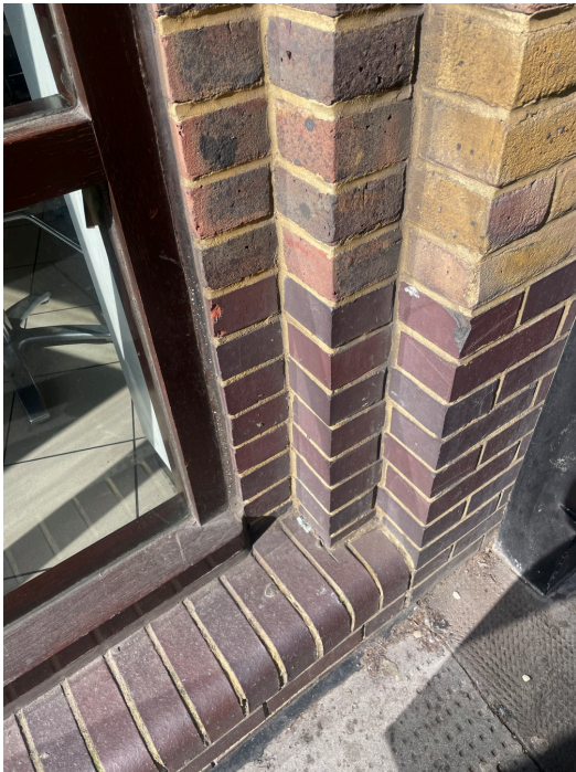
23.04.11 - Mercer Street elevation brickwork detail in window reveal and cill.
