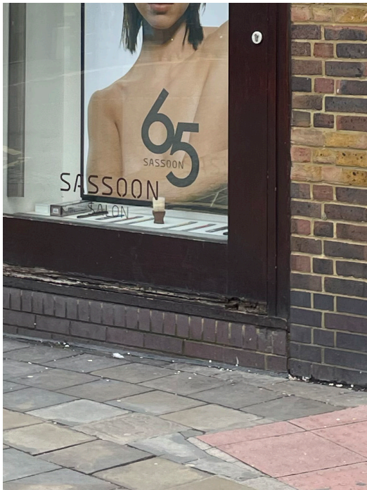
23.04.11 - Elevation facing onto Seven Dials. Detail of unoriginal brick upstand to form plinth for window frame. Brick not keyed into flanking original brickwork.
