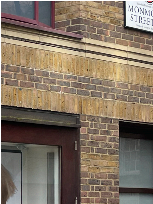
23.04.11 - Monmouth Street elevation. Detail of original brown brickwork with yellow London stock brick banding in soldier bond. Above brick a limestone band.
