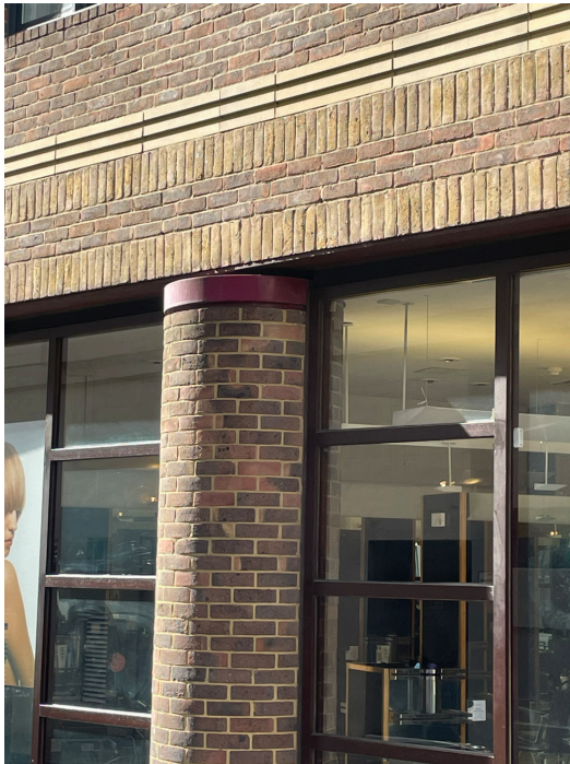
23.04.11 - Mercer Street elevation detail of cylindrical brown brick column with red-painted capital.
