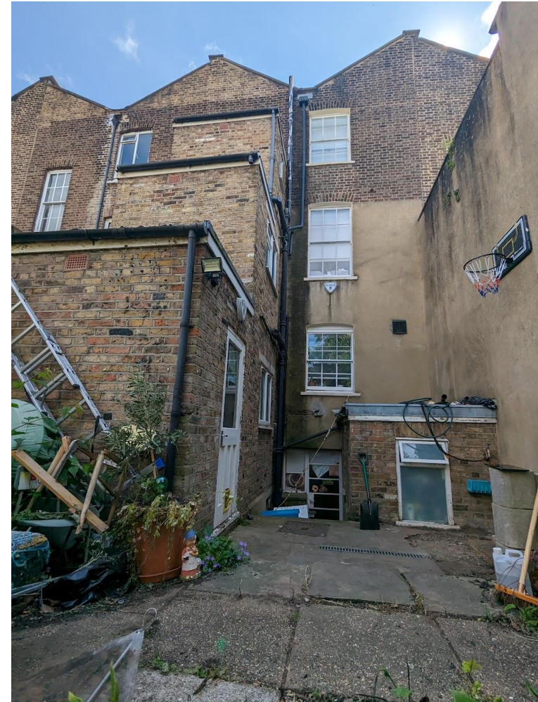
Image 2 – Photo of rear elevation
