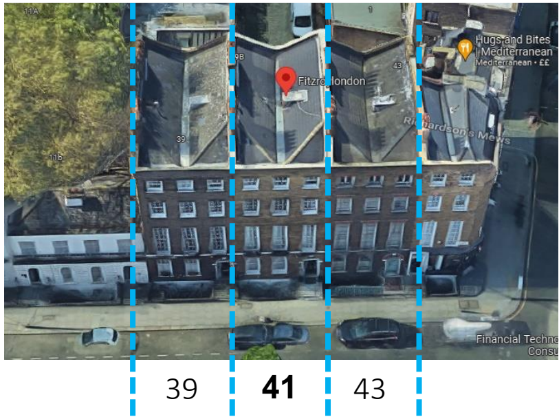
Figure 5- Roof view to front
