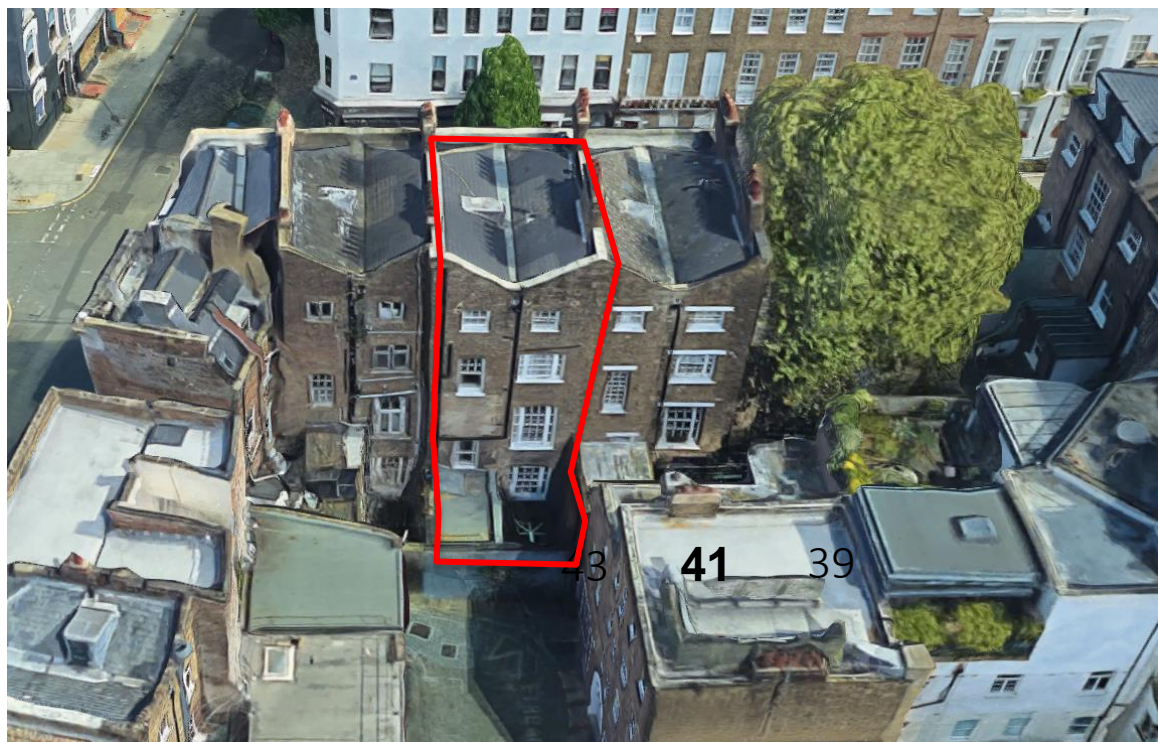
Figure 7- Rear view showing lightwell
