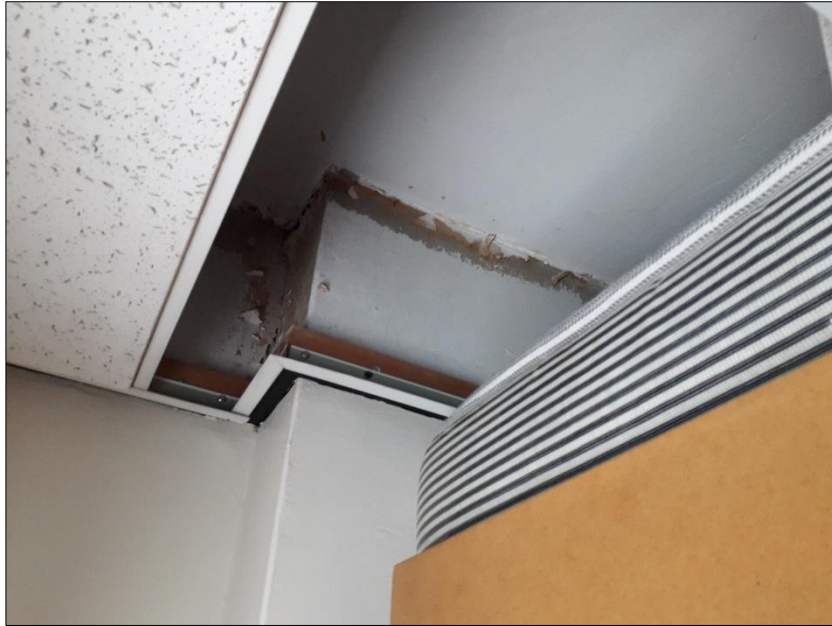
Photograph 8: indicative detail of second floor ceiling void showing plaster finish to soffit [03.04.2023]
