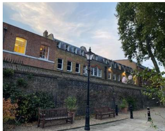
Figure 15 A view of the Jockey's Fields frontage from within Gray's Inn.
