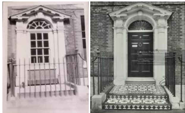
Figure 13 & 14: A blocked door at No. 5 Bedford Row (© CLSAC HS 524A date unknown) and after reinstatement in 1956 [LMA London Picture Archive 69432]
