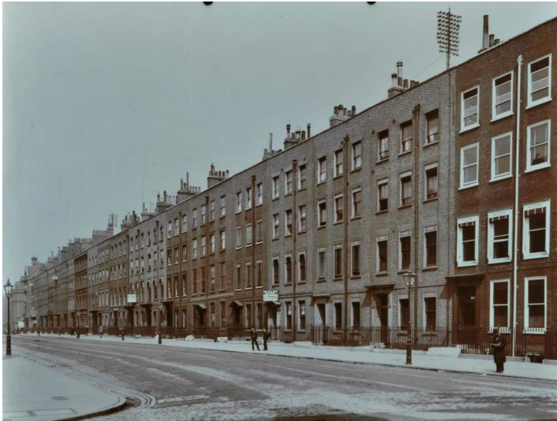
Figure 12: Nos. 2-20 Bedford Row in 1907 (Nos. 3-5 looking refurbished) [© LMA London Picture Archive 69572]
