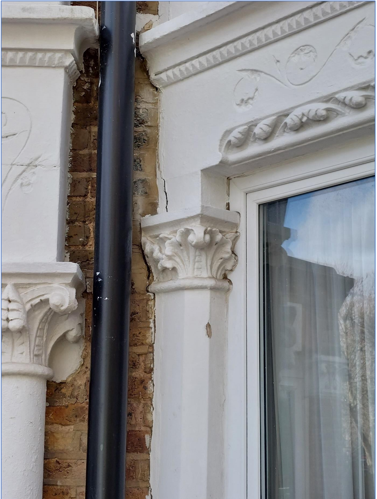
Photo 5: Cracks in window surround, claim address
