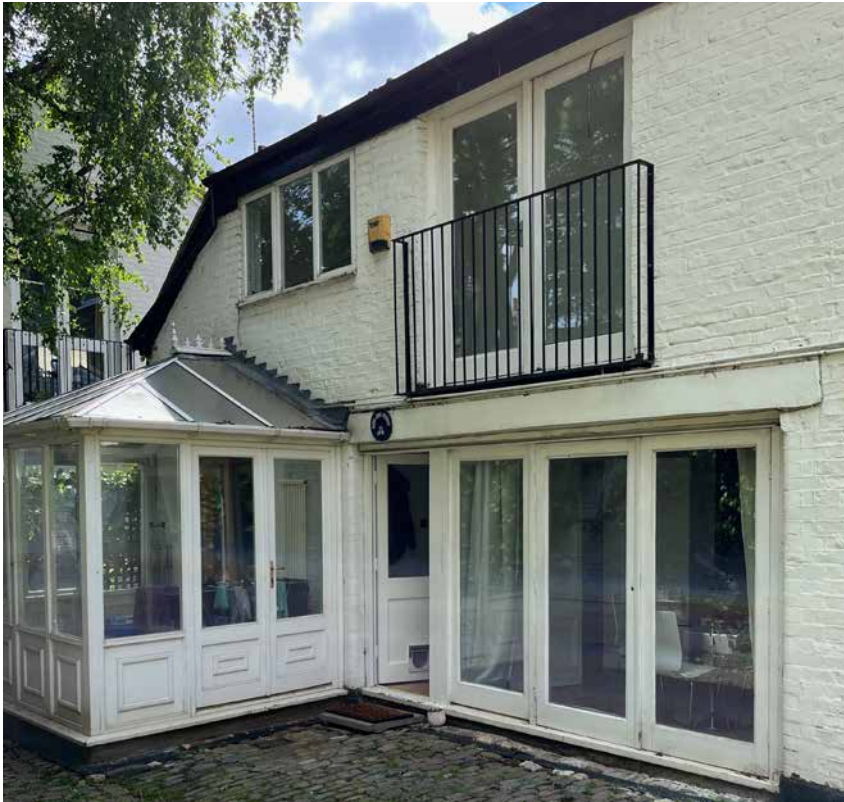
Image 01: 2 Falkland Place front elevation and entrance
