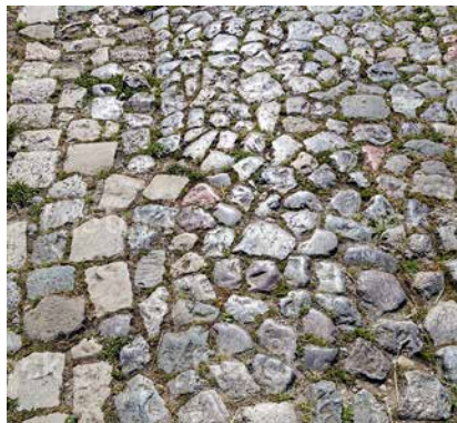
Image 05: Refurbished cobbled paving
