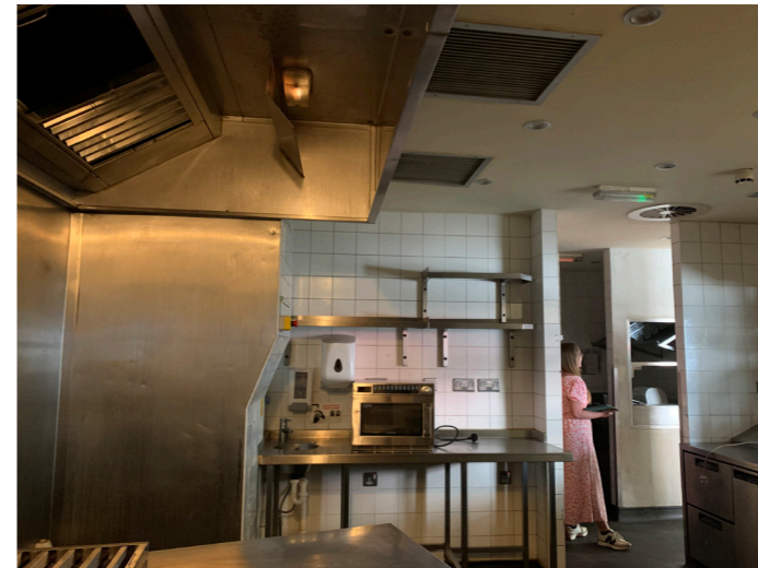
Figure 4.4 Interior of restaurant kitchen
