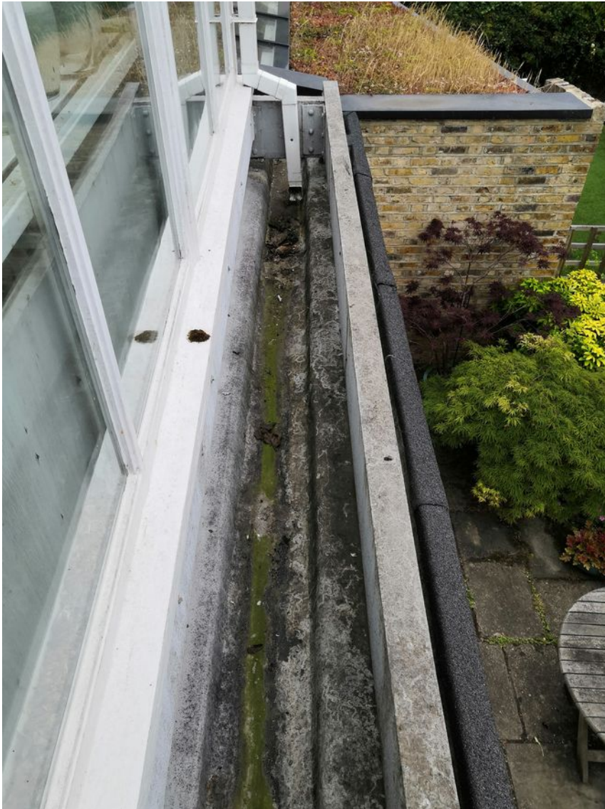
The rear facade of the conservatory showing the exposed timber support structure and concealed gutter.
