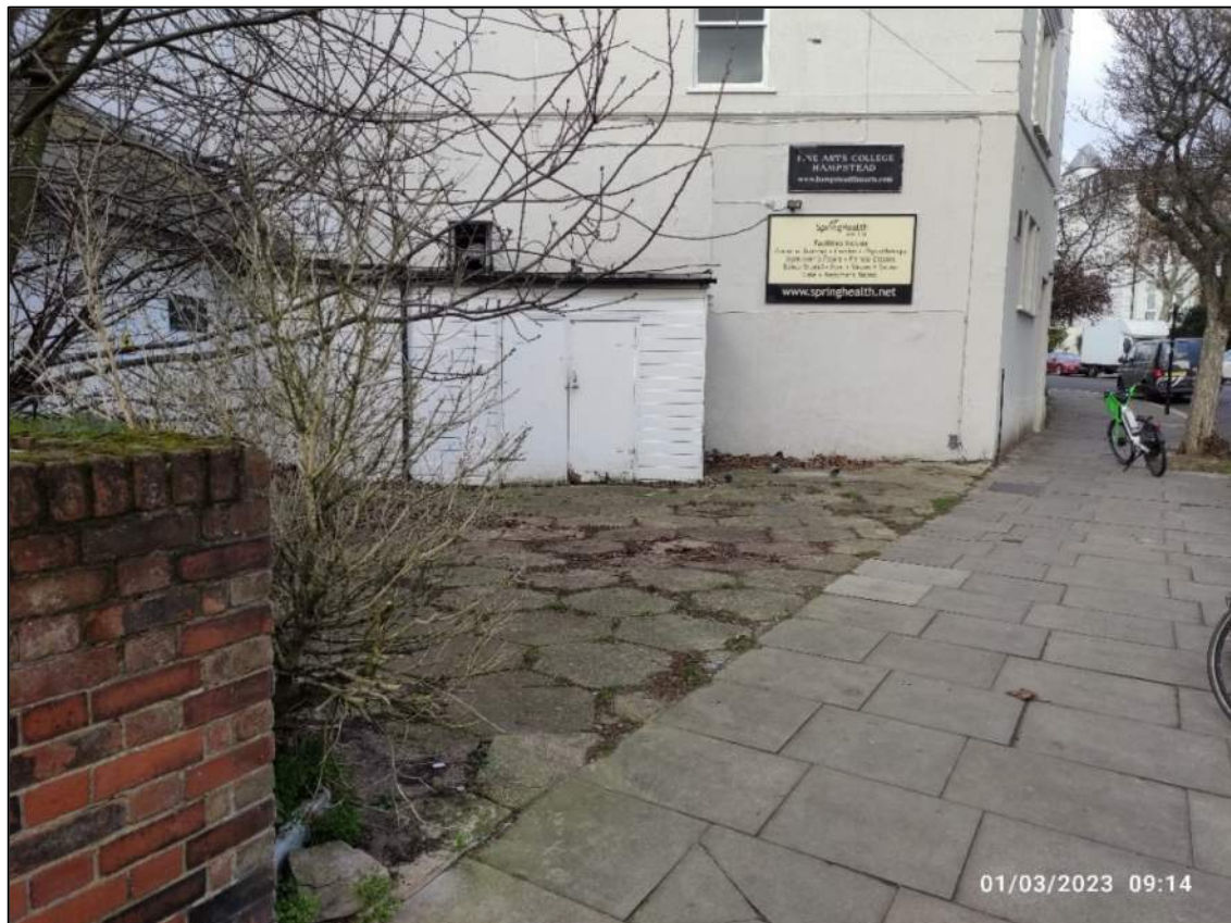
Figure 5.1 Existing access and forecourt
