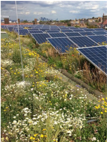
Fig.2: Green Roof (Biosolar)
