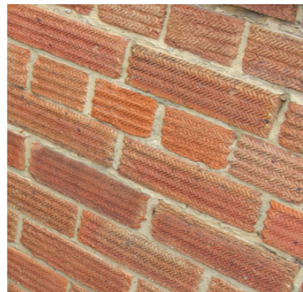
Fig. 1: Cleaned existing bricks
