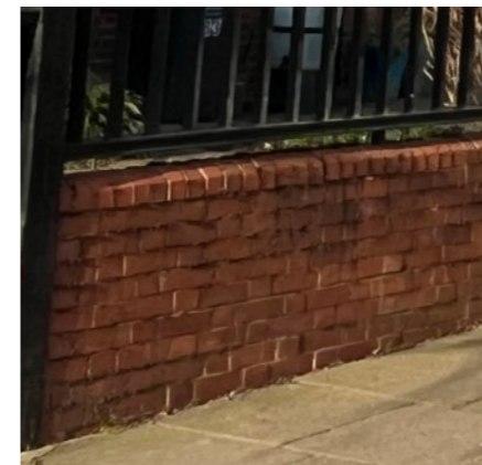
Fig.2: Proposed red brick (flemish bond , lime mortar)
