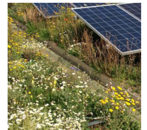
Fig. 8: Green roof + PV's
