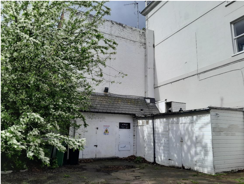
Photograph 1: Hardstanding, Building 1 and semi-mature cherry tree – u1b and u1b5
