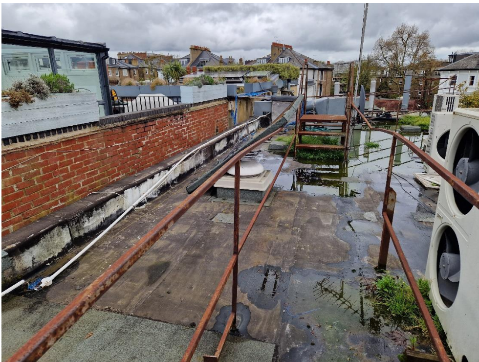
Photograph 2: Building rooftop, facing north – u1b5
