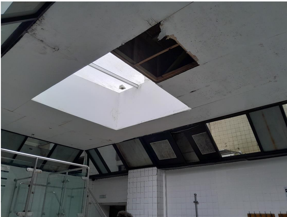
Photograph 8: Internal void spaces accessible by skylight (Target Note 3, Figure 1)
