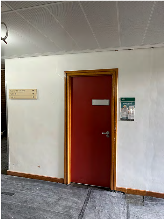
IMG_7320 Rm 482 later addition
