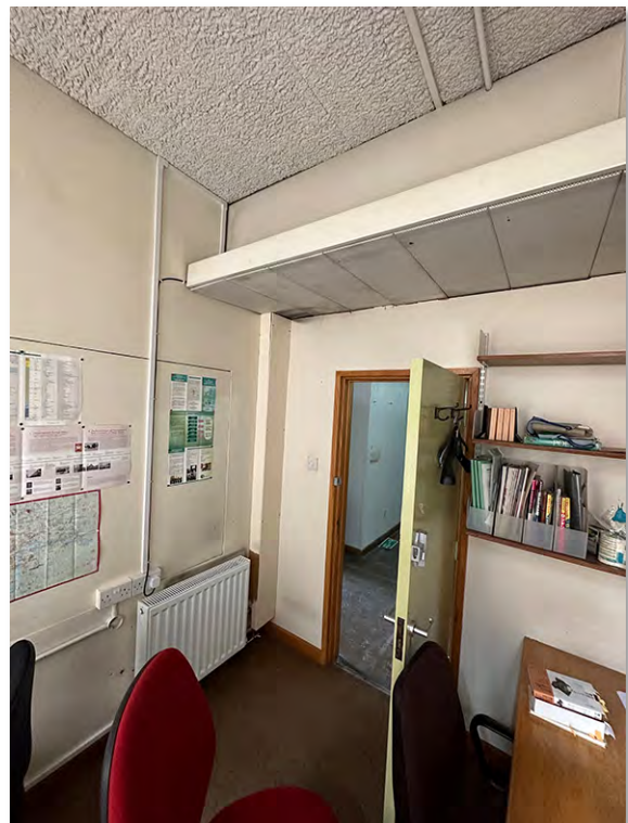
IMG_7291 Rm 349 Interior showing dropped bulkhead, with soffit
