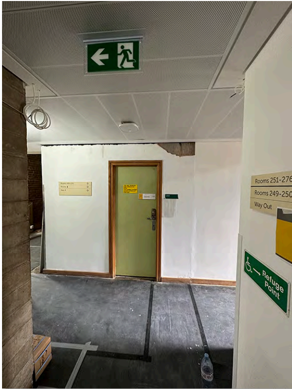
IMG_7259 Rm 249 later addition
