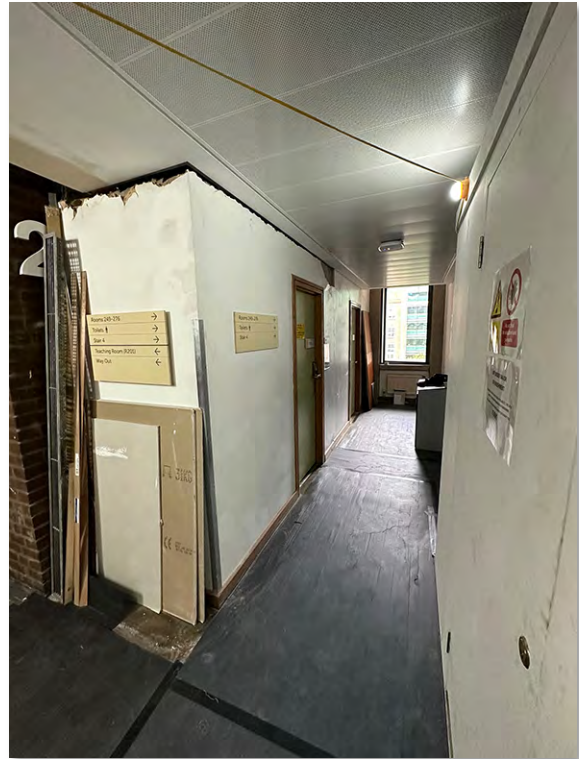
IMG_7260 Rm 249 later addition
