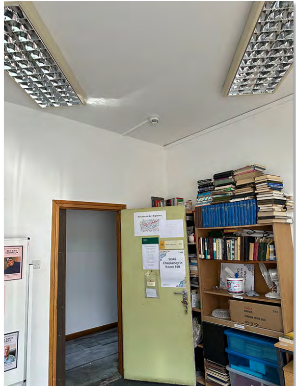
IMG_7469 Interior Rm 350
