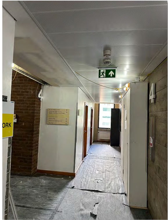
IMG_7321 Room 482 later addition
