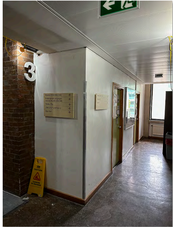
IMG_7284 Room 349 later addition
