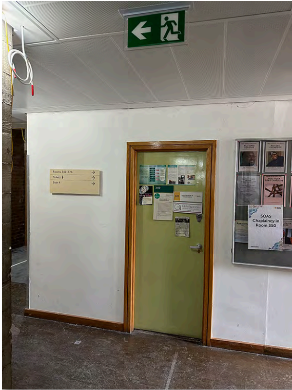
IMG_7285 Rm 349 later addition
