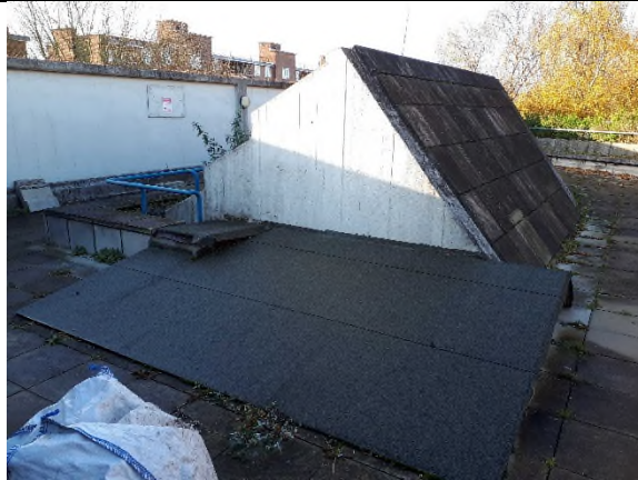
19. TRA Hall – Roof terrace – Area to centre ‘Skylight’ to TRA hall below and felt and timber covering in foreground.
