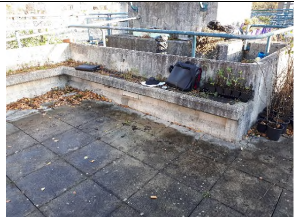
9. TRA Hall – Roof terrace – Main area showing built seating and irrigation sump and channels beyond around presumed water tank housing
