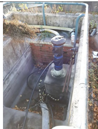
24. TRA Hall – Roof terrace – Recessed water channel and sump with irrigation pump (broken) housed in brickwork
