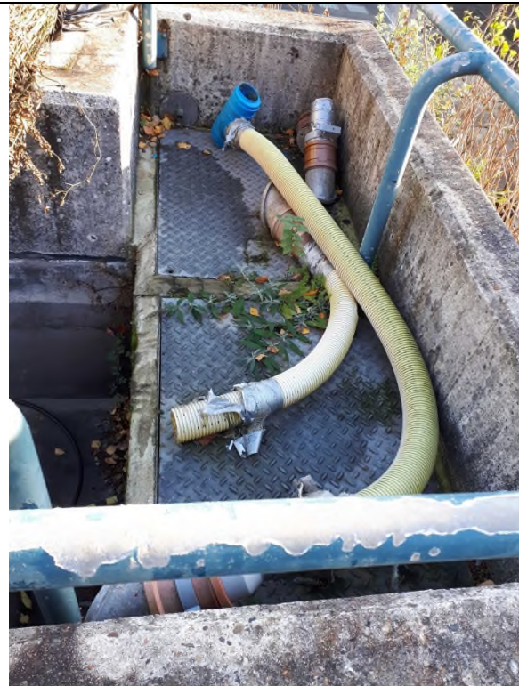
28. TRA Hall -Roof terrace - Access hatches to side of sump and plastic pipework
