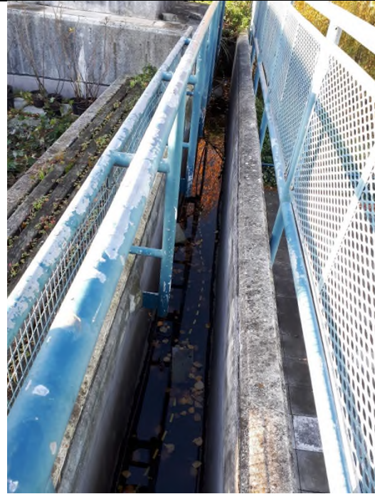
26. TRA Hall – Roof terrace – Recessed channel for rainwater discharge from roof linked to sump
