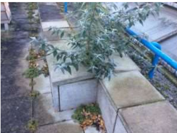
Vegetation growth likely to be penetrating waterproofing allowing water ingress.
