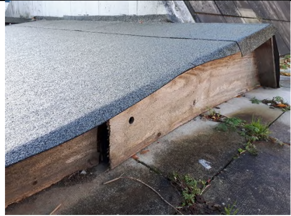
20. TRA Hall – Roof terrace – Felt and timber covering by ‘Skylight’ detail
