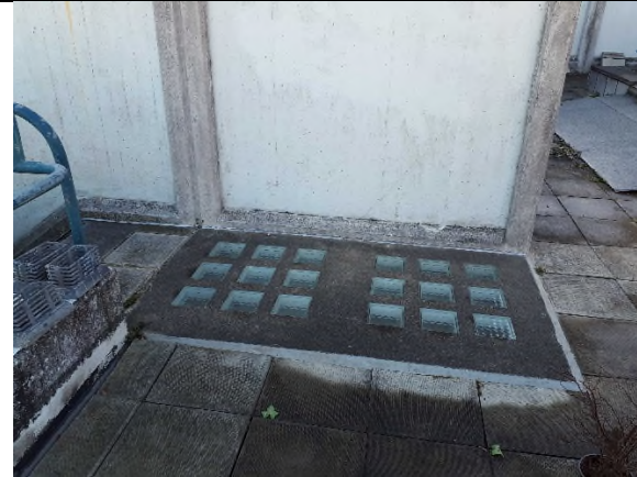
7. TRA Hall – Roof terrace – Pavement light
