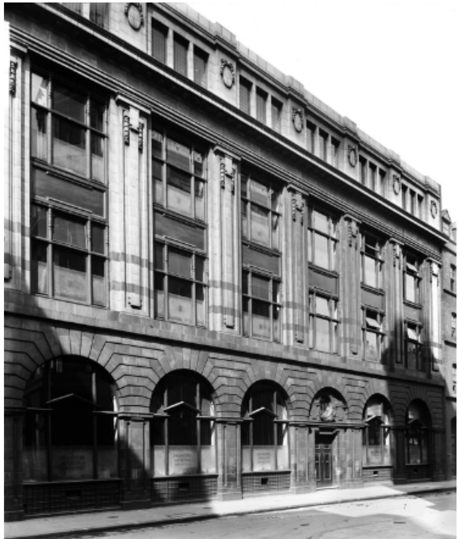
Figure 8: The Brooke Street elevation of the Prudential Assurance Co. building, August 1919
