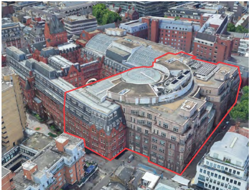
Figure 18: View looking south-west in 2021, with 2 Waterhouse Square outlined in red
