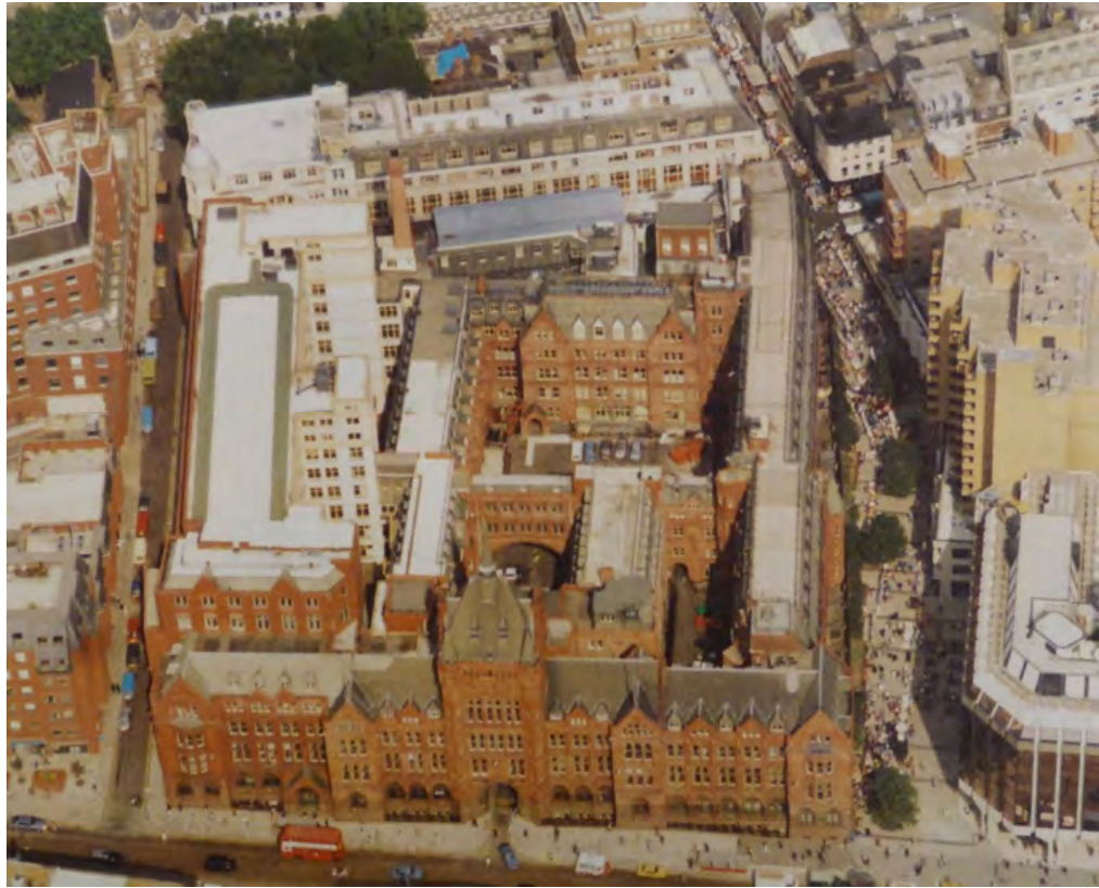
Figure 14: Aerial view looking north, c.1988
