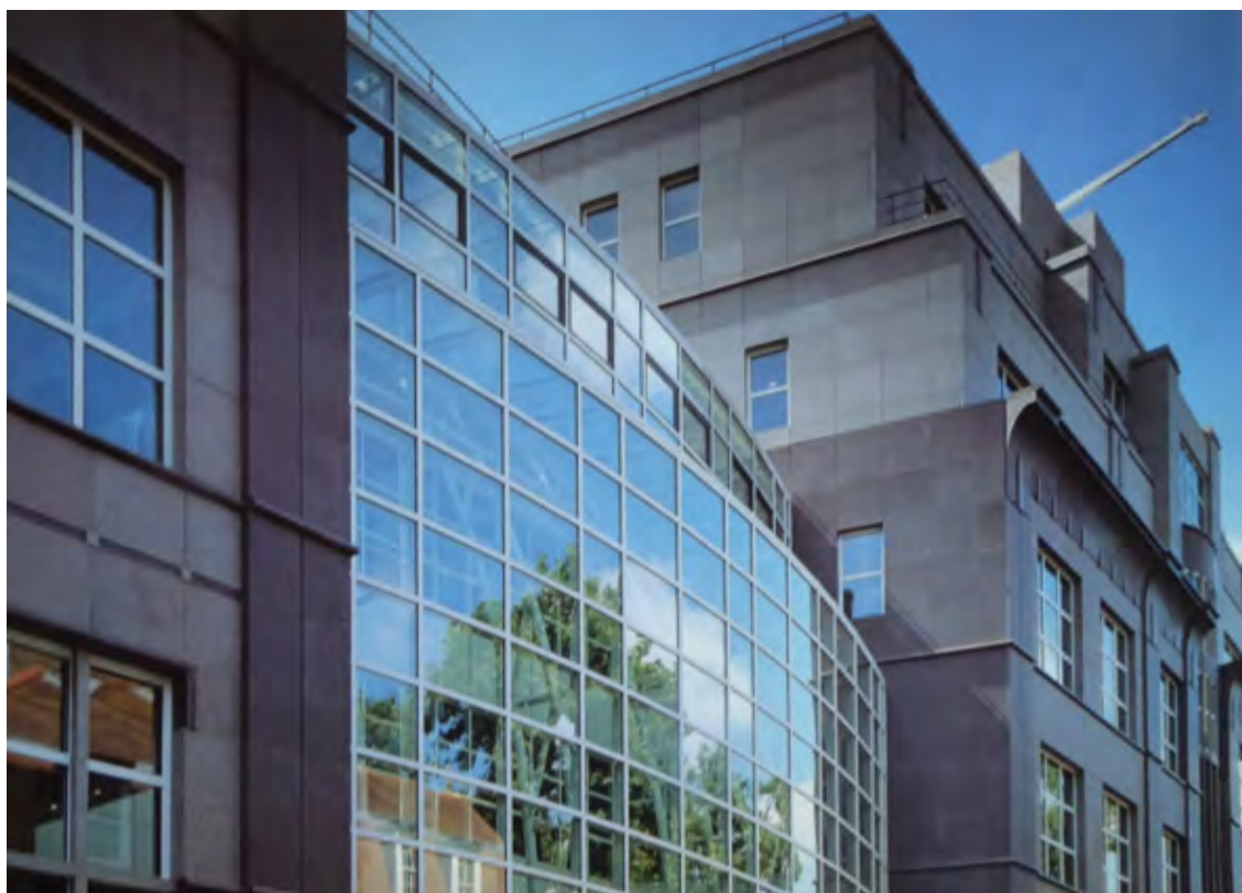
Figure 21: Beauchamp Street elevation of the North Court (2 Waterhouse Square) showing glass-walled atrium and set-back upper storeys
