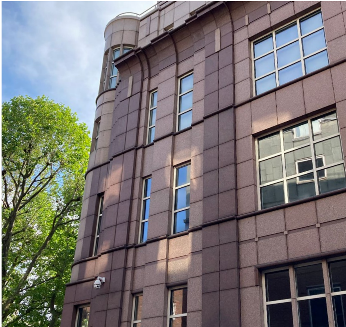
External Granite cladding on 2 Waterhouse Square
