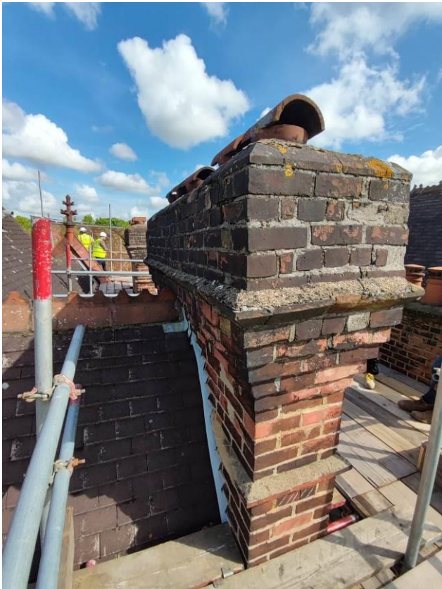
Plate 8: Rear view of rear stack leaning against the roof
