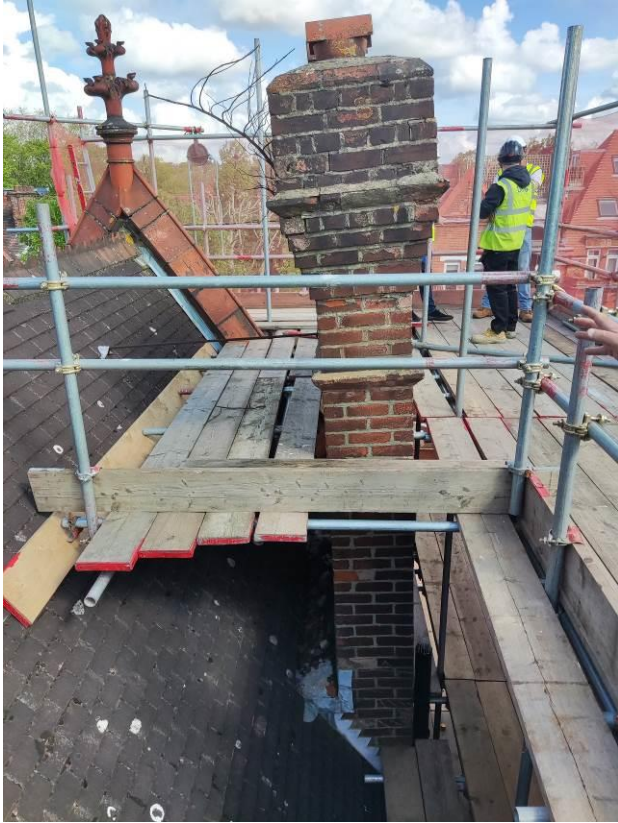
Plate 3: Top section lean is more pronounced.
