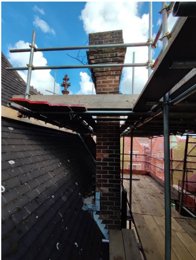
Plate 2: View of front stack leaning towards the building
