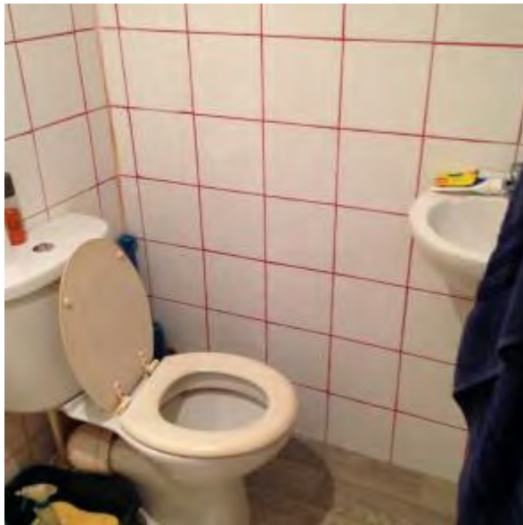
Studio bathroom (unrefurbished)
