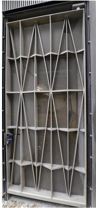
Figure 3 – Existing Plant Room Door to be Replicated
