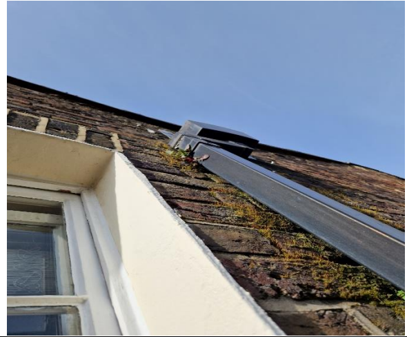
Rear elevation down pipe.
