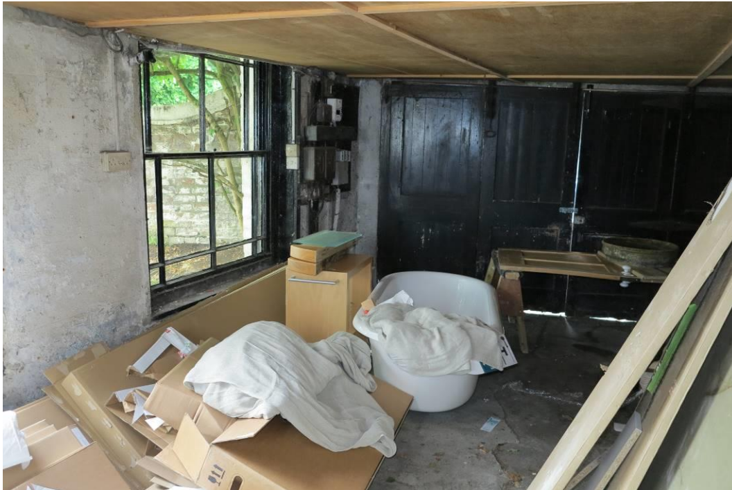
Plate 7. A first floor has been inserted in the garage/coach-house, cutting across the window openings
