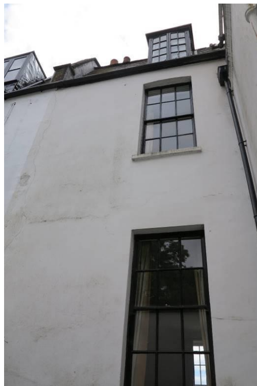
Plate 2. Original window openings on the rear of this and other of the Holly Terrace properties tend to have a slightly-cambered head
