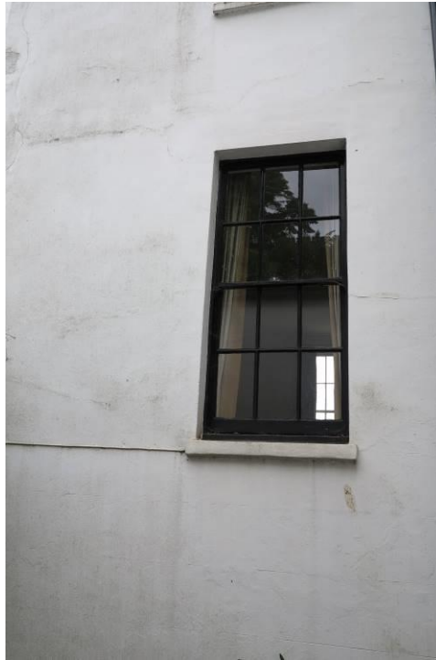
Plate 1. The ground-floor window opening to the eastern bay on the rear elevation is a modern insertion or reinstatement
