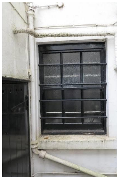
Plate 1. Closet wing window to be converted to doorway in rear lightwell
