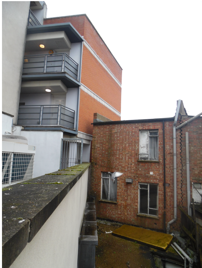
PH4 - REAR VIEW OF No 7
