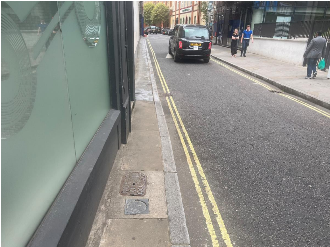
Figure 5-3: Key Route 1 – Worst Point – Parker Street Southern Footway
