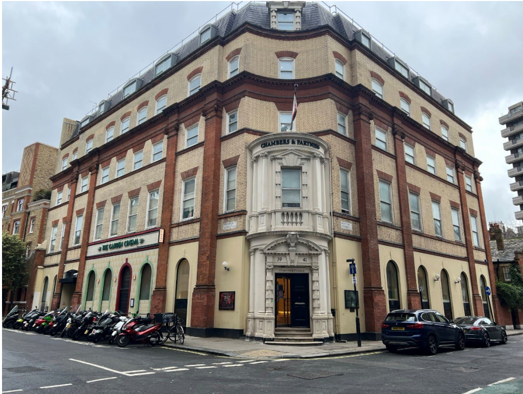
Figure 2. Main entrance at 39-41 Parker Street
