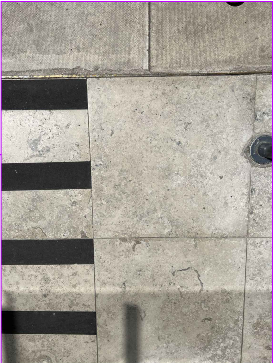
NEW LIMESTONE PAVING WITH NON SLIP BLACK INSERTS TO MATCH
