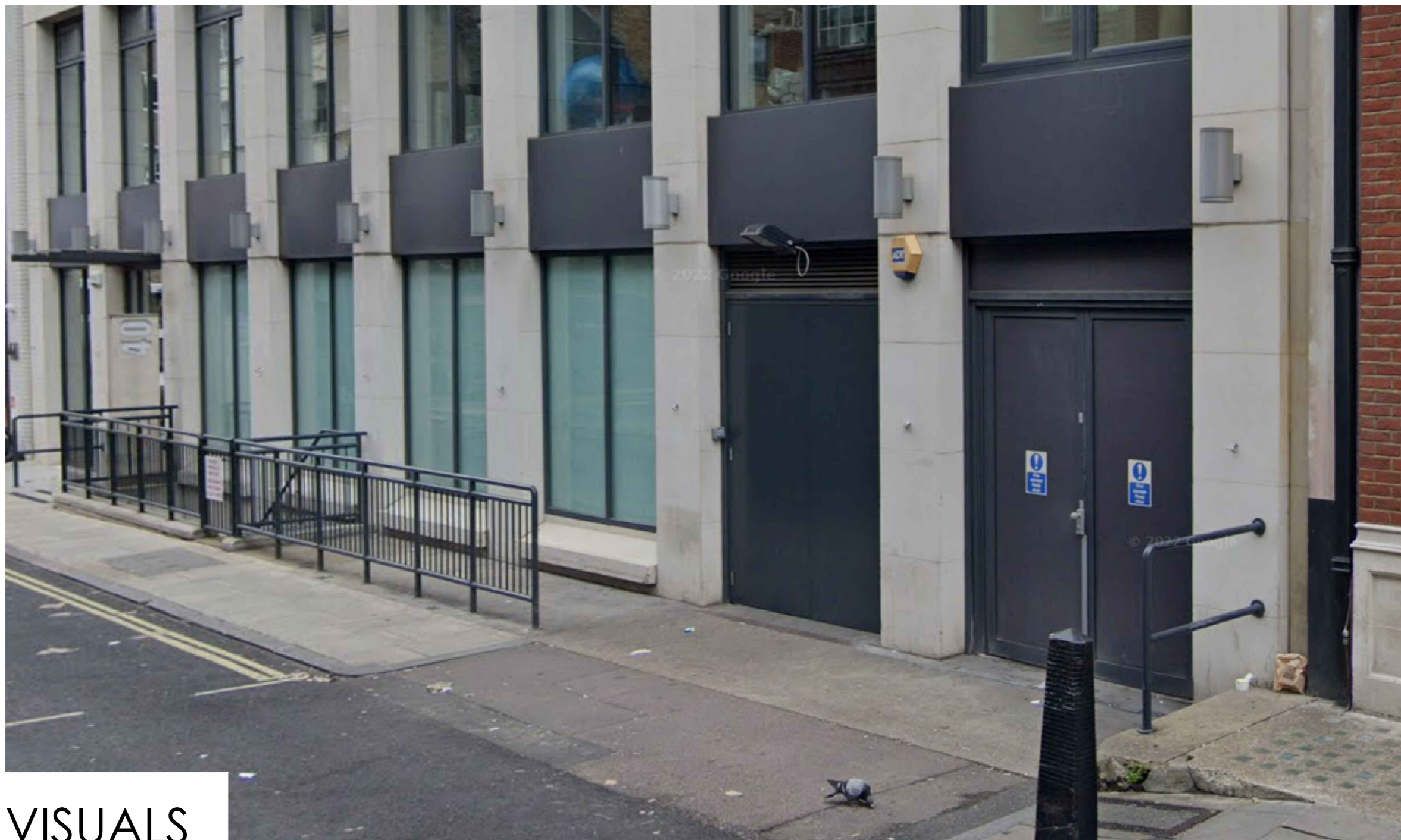
Existing street view
