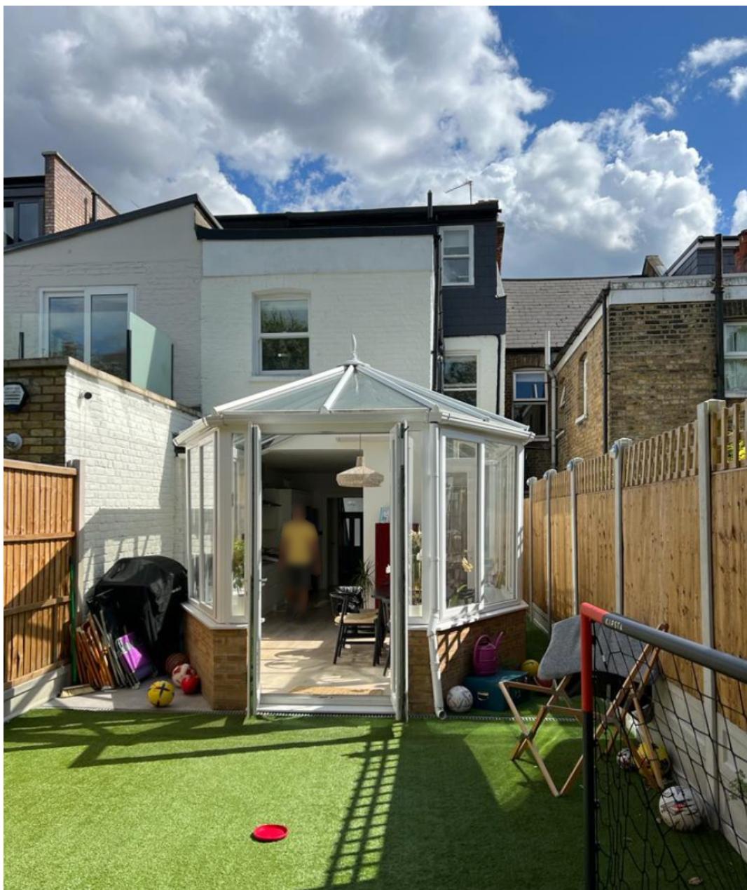
38 Ingham Road existing rear
