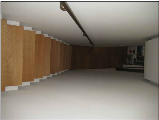
New stairs to attic Solid oak on timber/Plasterboard construction
