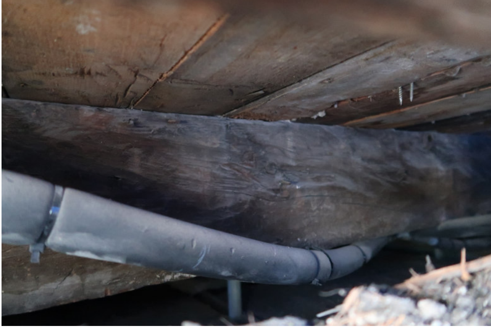
Floor beam behind.
