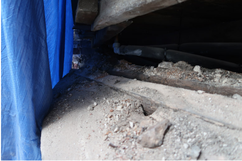
Three timbers at front of bay.
