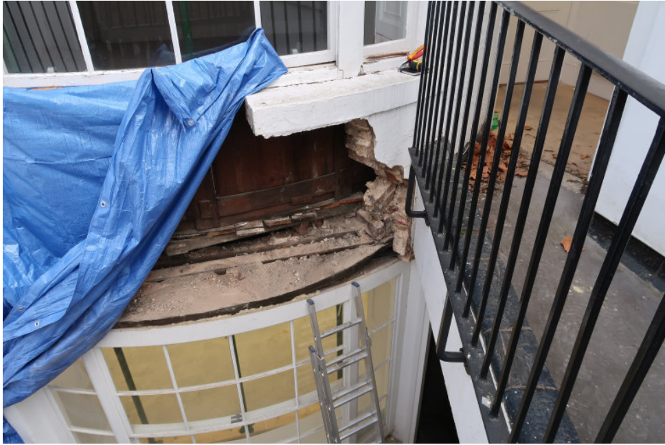
View from ground floor.
