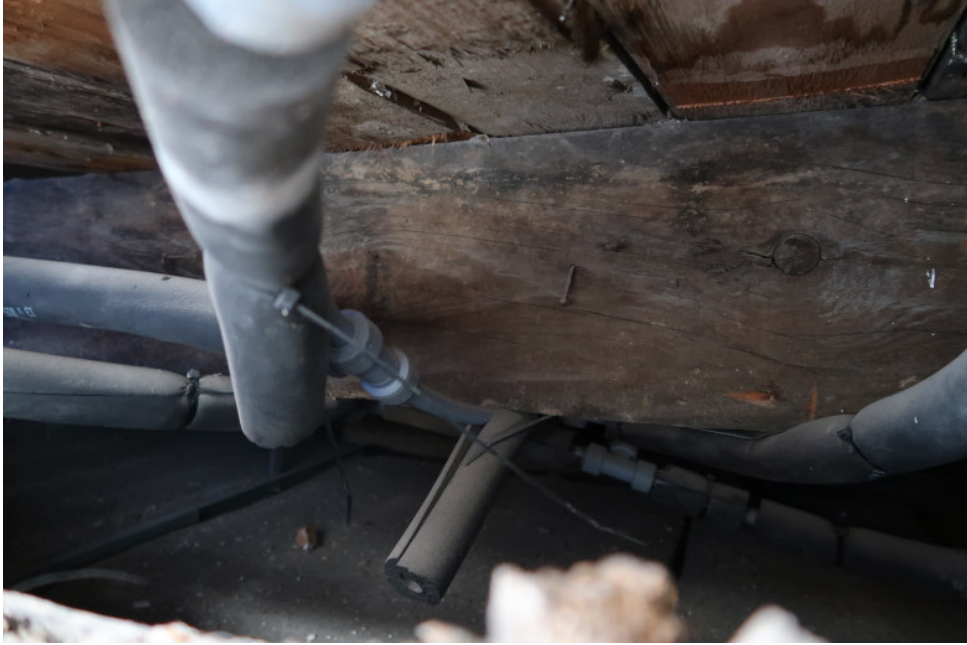
Floor beam towards rear of bay.
