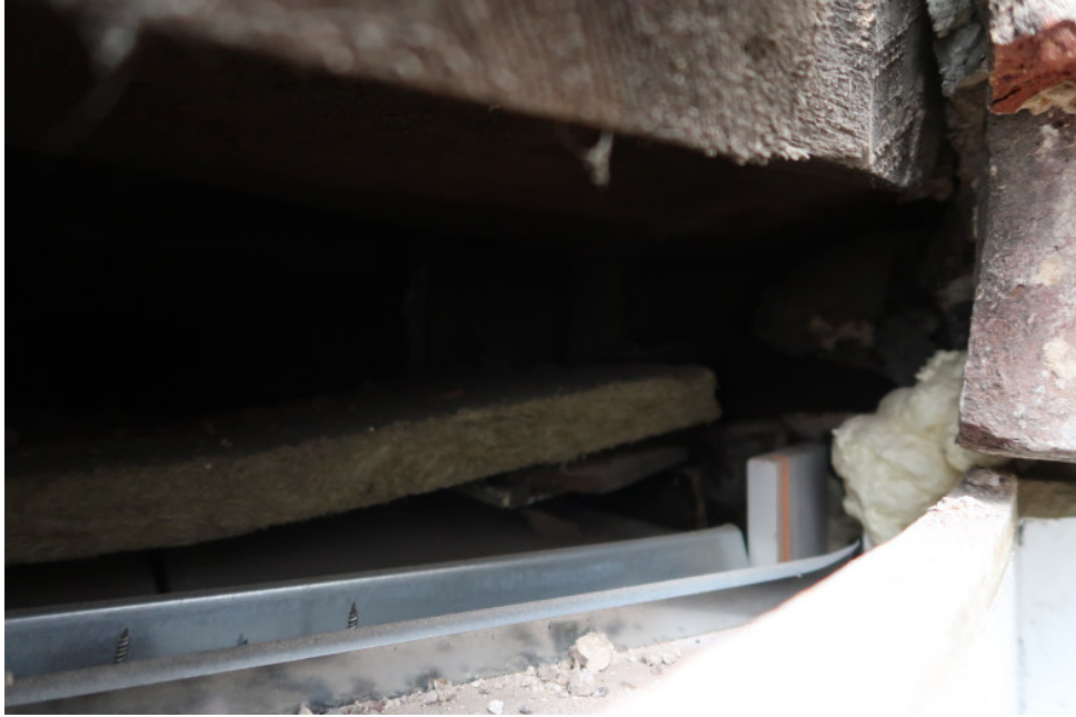
At RHS support.
