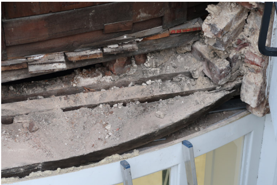
Three timbers at front of bay.
