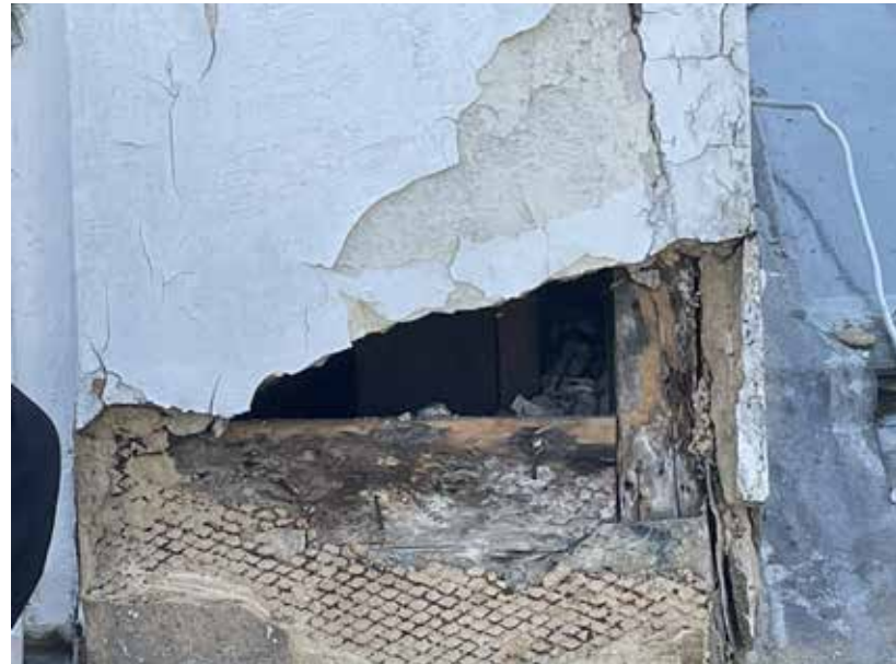
Image 9: render damaged - base north west corner of cupola
