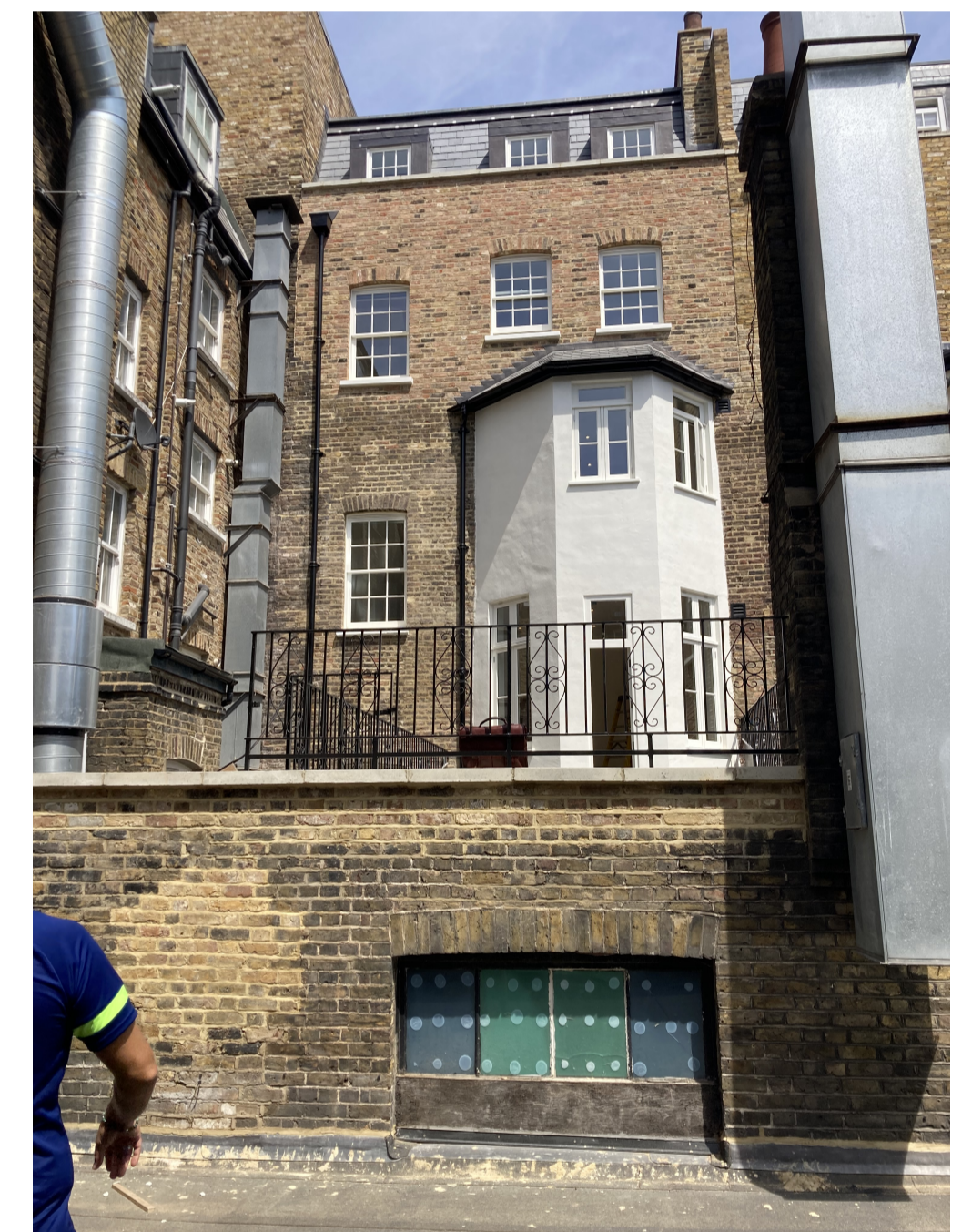
Image of existing blocked off opening - to be retained as it.
