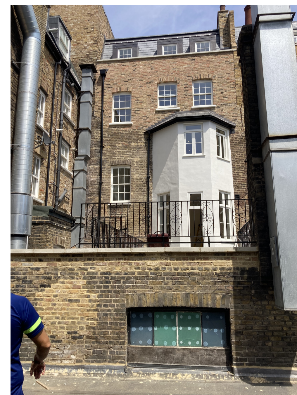
Image of existing blocked off opening - to be retained as it.
