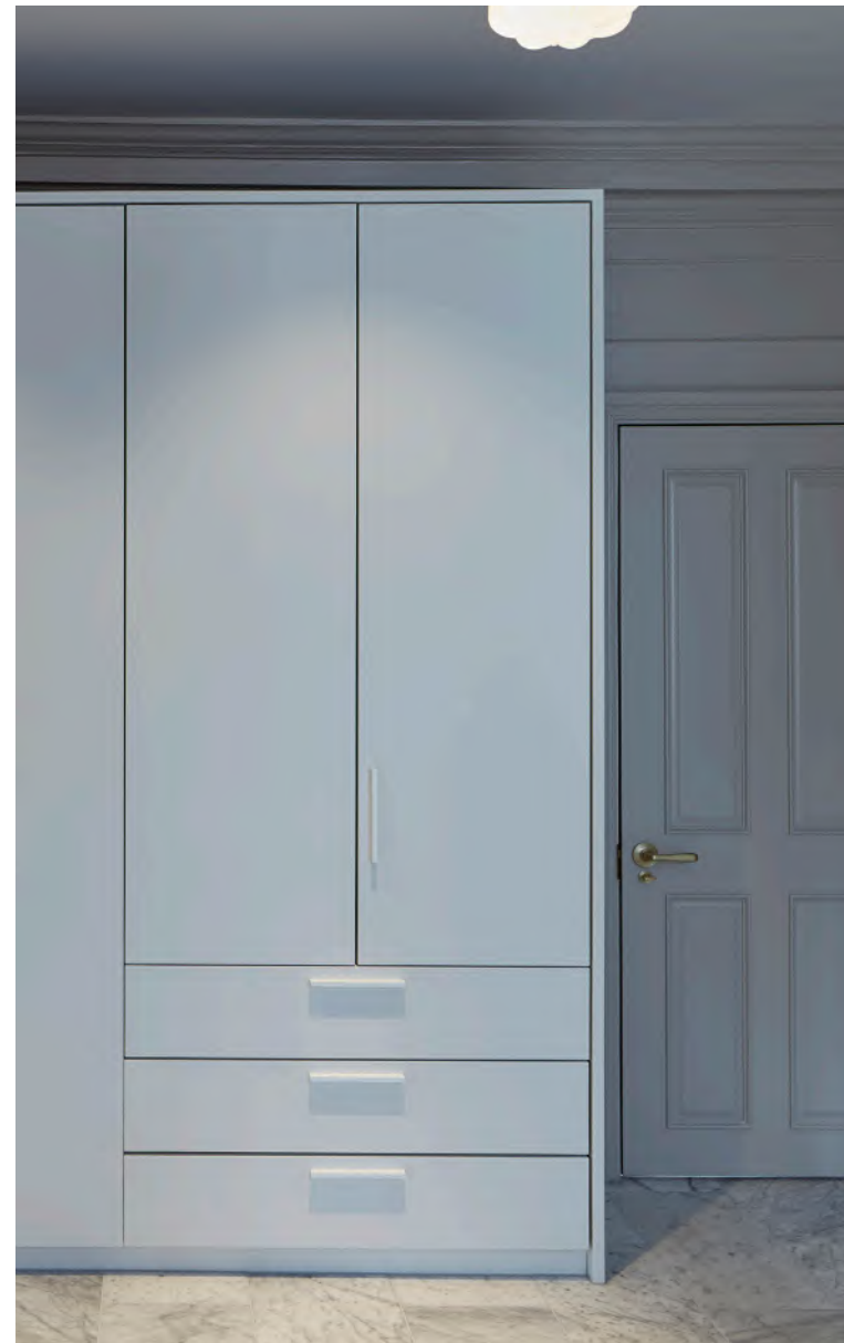
Example of joinery designed so that panelling and cornicing remain in place, 36 Great James Street by Quinn Architects
