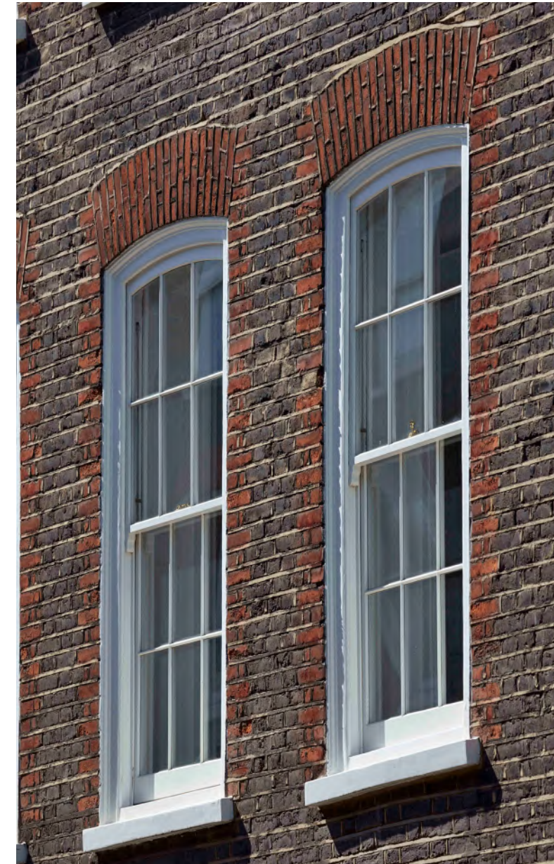
Sashes and sash boxes refurbished
