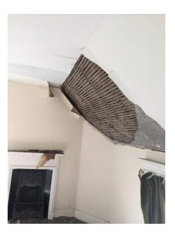
Photo 9: Internal damage to the ceiling on the second floor, showing the construction of the roof – no access point
