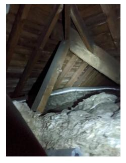
Photo 10: The loft void was well-sealed and recently re-insulated
