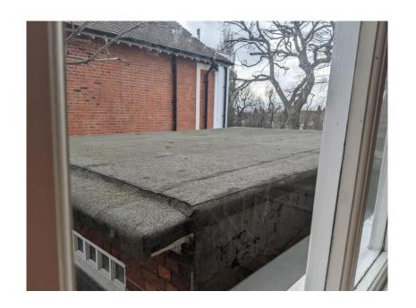
Photo 3: Flat felt roof covering the rooms over the garage on the southern side of the existing building
