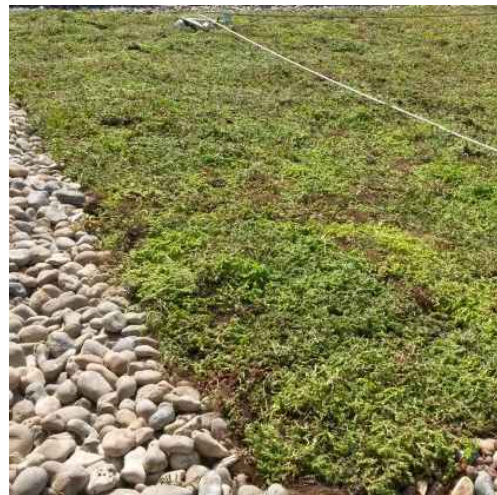
11 - Roof Covering * Sedum Vegetation Blanket
