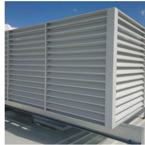
09 - Louvre Plant Screen * PPC Aluminium RAL- RAL 7035
