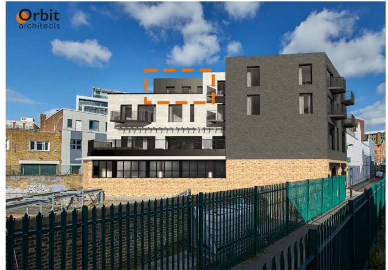
CGI view of propose design from railway bridge. Third floor extension to be zinc standing seam.
