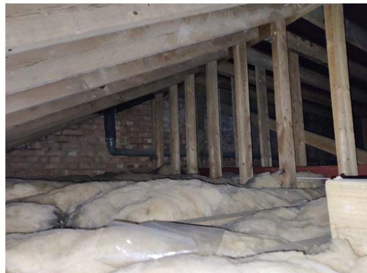
Existing insulation at ceiling level - no insulation between joists
