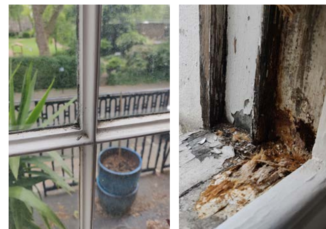
Existing window bars and visible frame deterioration
