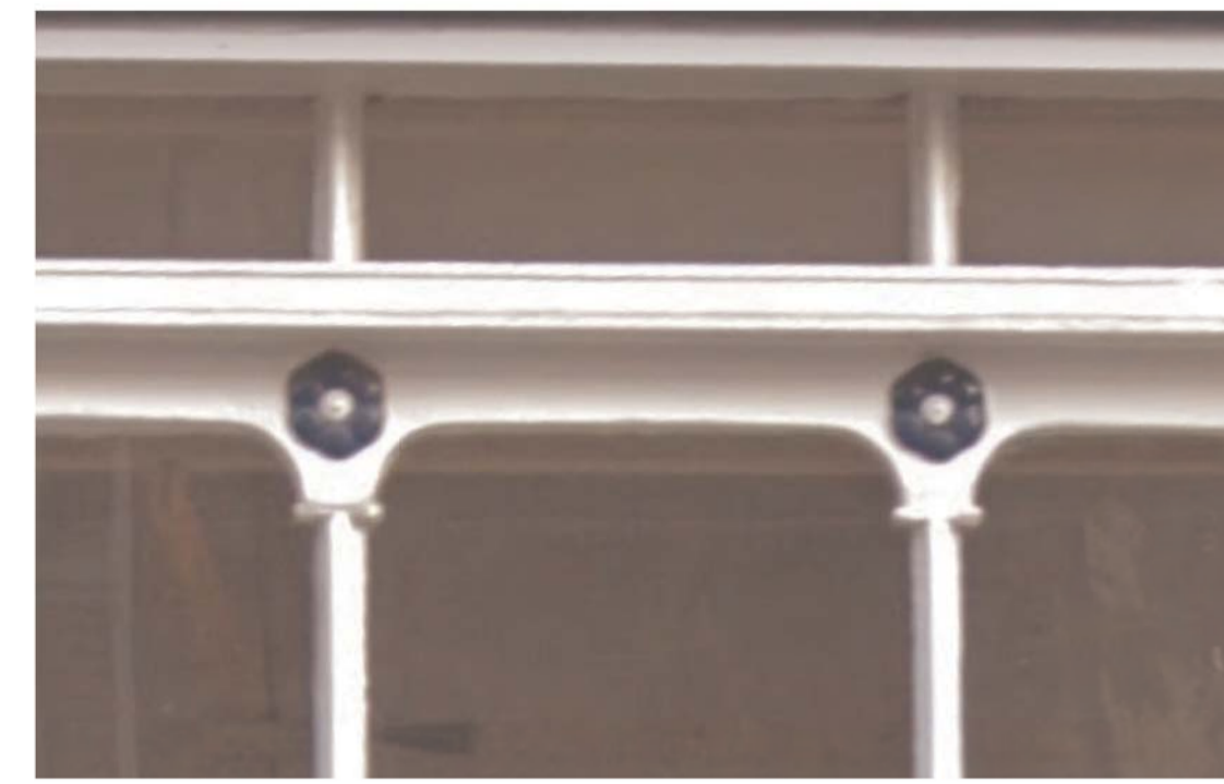
Detail 01 Original decorative flower detail to be carefully removed from existing shop-front window and fixed to new window frame
