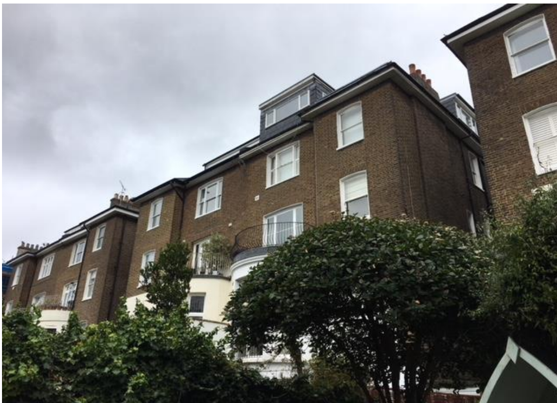
Above: The rear view of No.27
