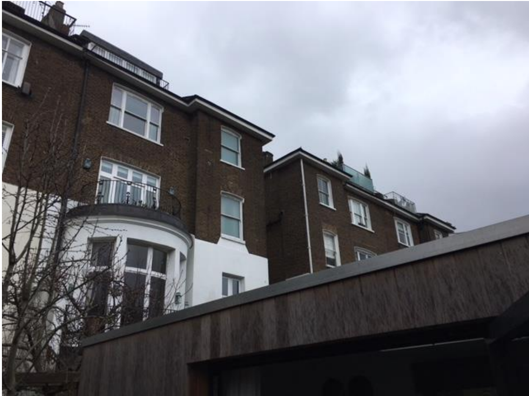
Above: The rear view of No.31
