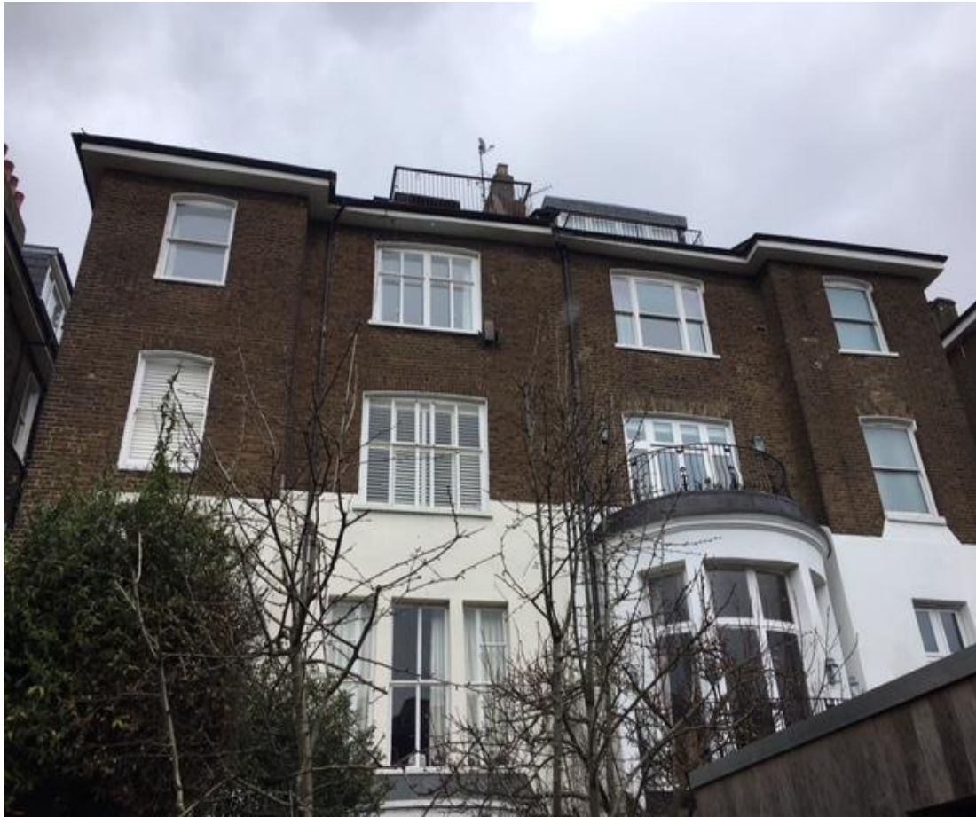
Above: The rear view of No.29
